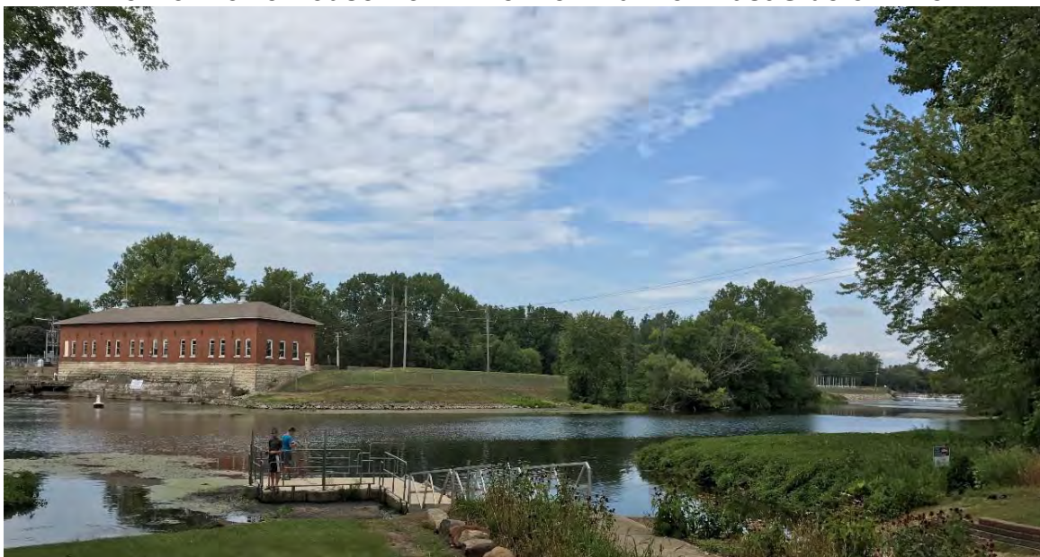
Photo 5.9-1 View of Powerhouse from Riverview Park on East Side of River
